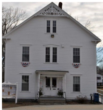
Town Offices Phillipston
