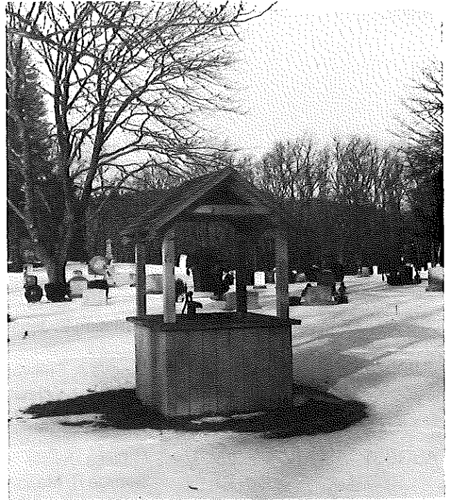
New Well House in the South Cemetery.
